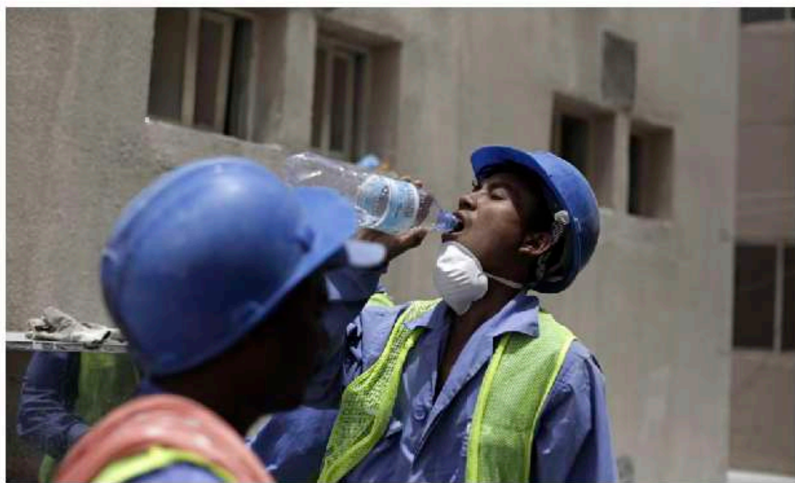
📷 A Nepalese worker takes a break during a government-organised media tour of World Cup construction projects. Photograph: Maya Alleruzzo/AP
